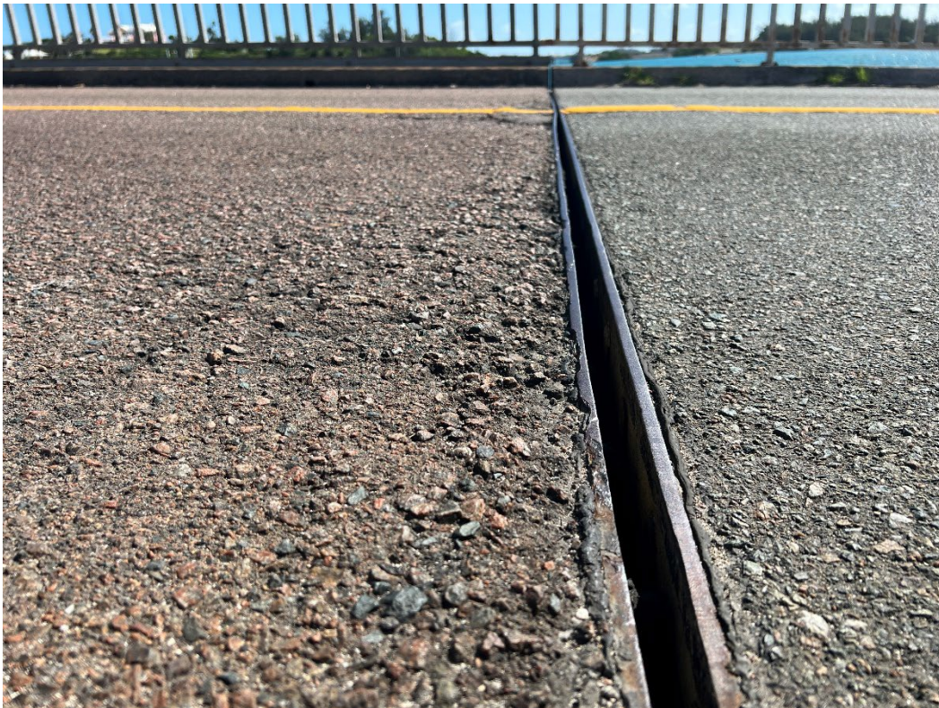
Photograph 1 – Existing end plates
