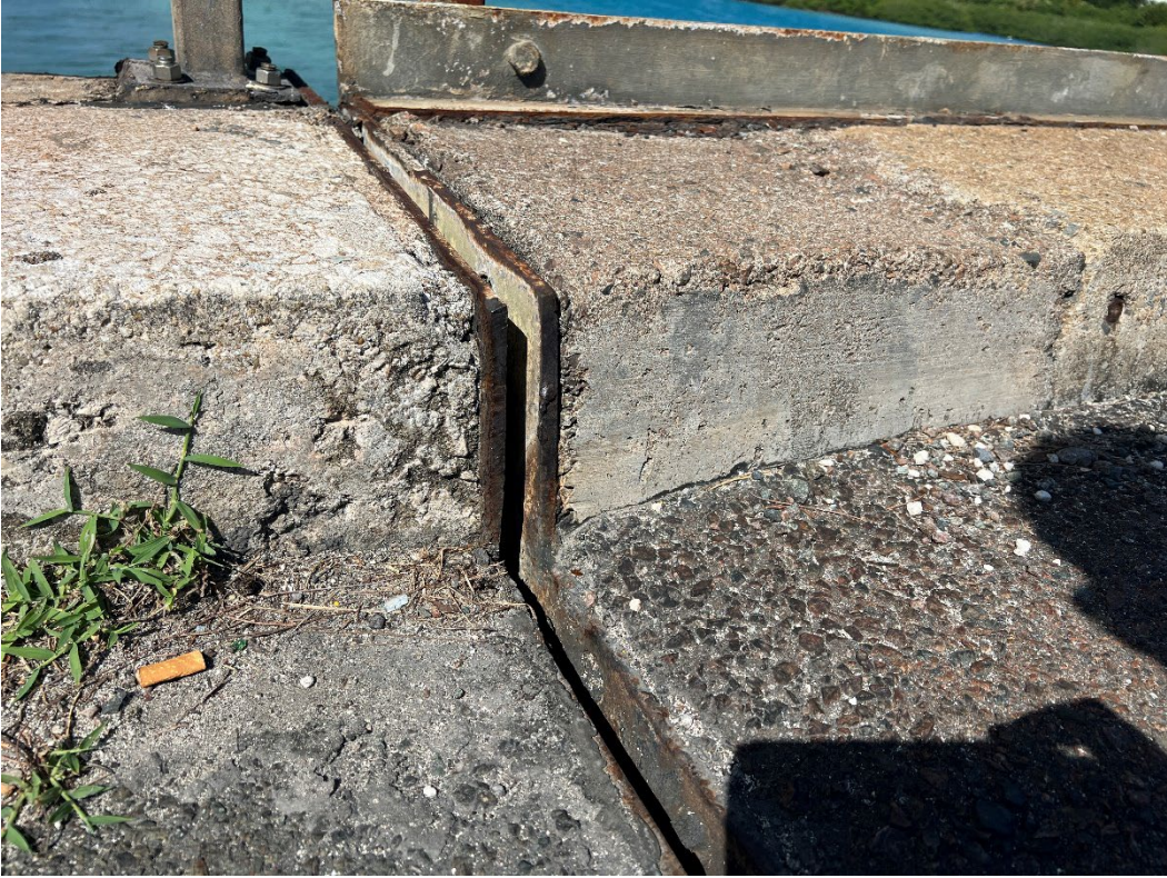
Photograph 2 – End plate at curb location
