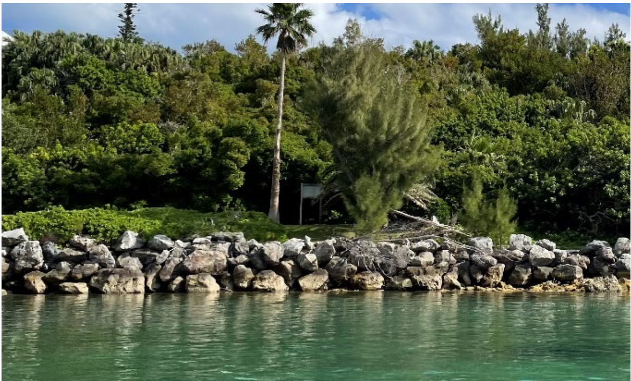
Figure 10.15 Somerset bridge (top) and rock revetment adjacent to bridge (bottom)
