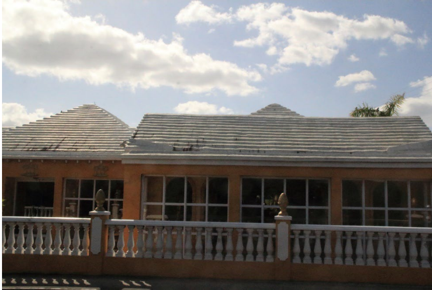
Limestone tile roof top with guides to channel rainwater to storage
