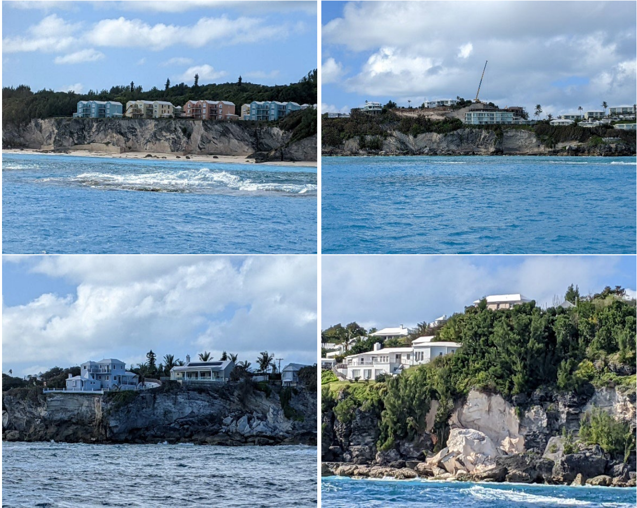
Figure 10.9 South Shore cliff failure
