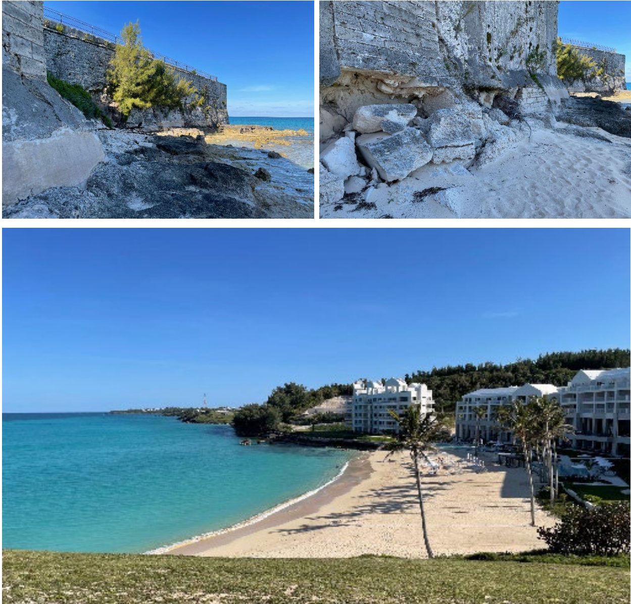
Figure 10.11 Fort St Catherine's eroding seawalls (top) and the Residences at The St Regis (bottom)
