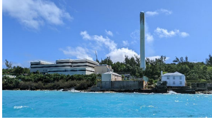
Figure 10.5 Desalination plant at Tyne's Bay
