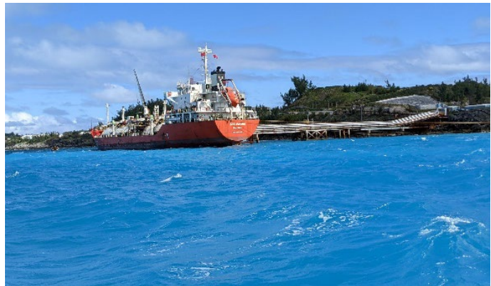
Figure 10.6 Sol Fuel Jetty
