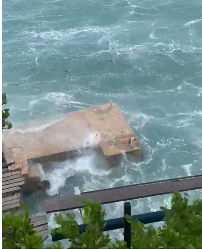
Figure 3.20 Wave conditions in Harrington Sound during Hurricane Flora when it was approximately 100 nm NW of Bermuda on September 23, 2022. Waves are seen to overtop the concrete dock, with wave height estimates of approximately 0.6m (2 ft). Image credit: Nick Strong/Mandy Shailer.
