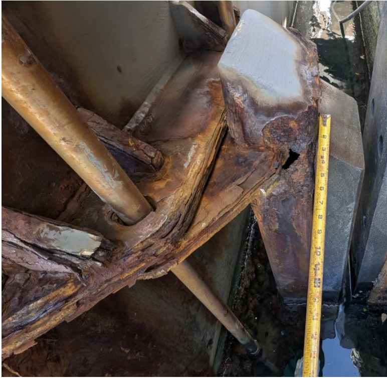
Wall Fender Failed Connection - South
