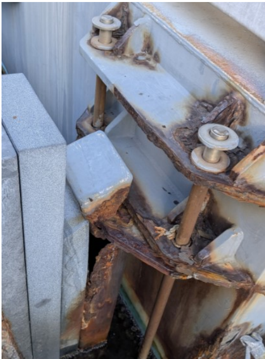
Wall Fender Failed Connection - South
