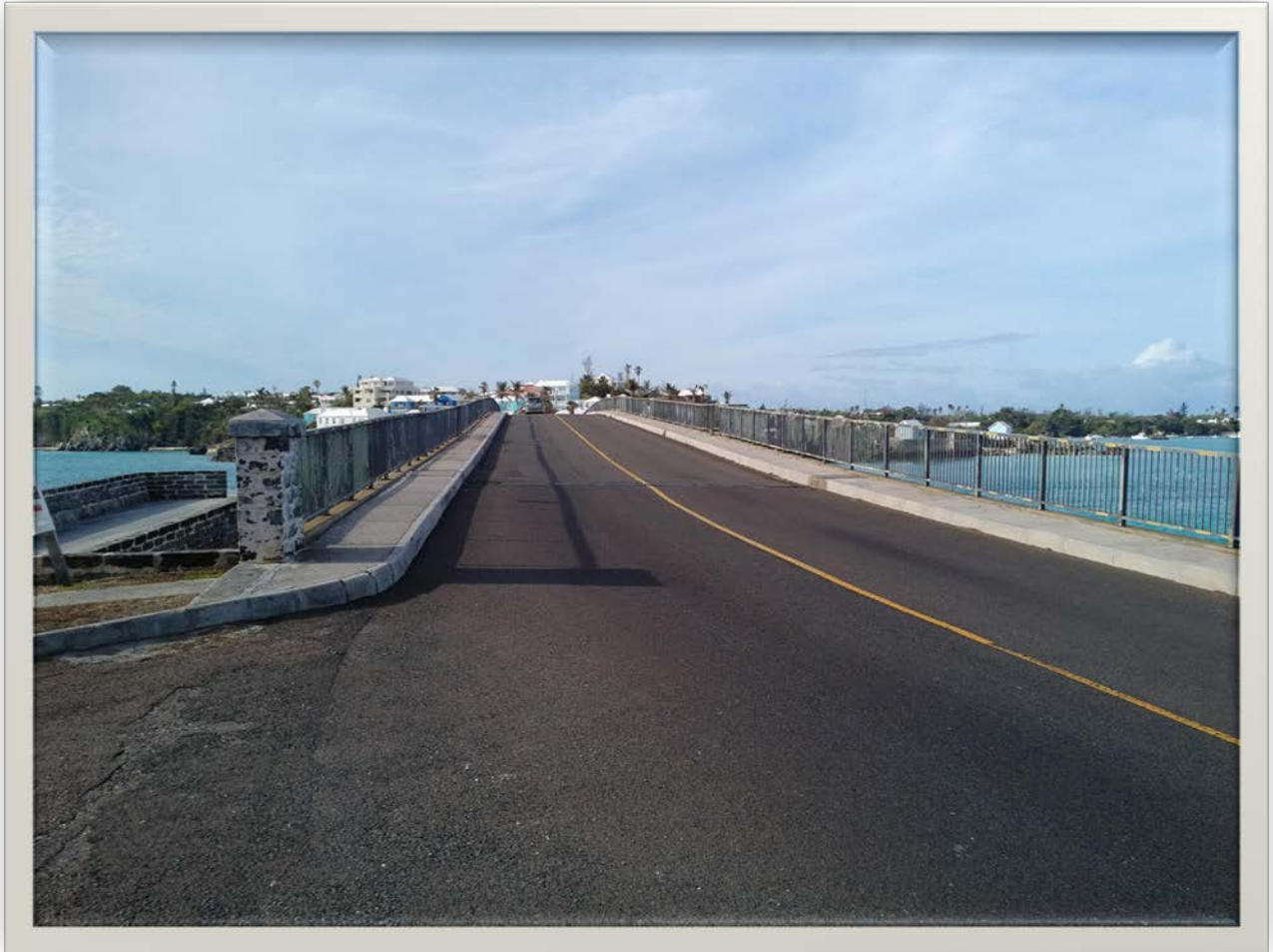
Figure 2: Watford Bridge Looking South, Handrails to be Painted
