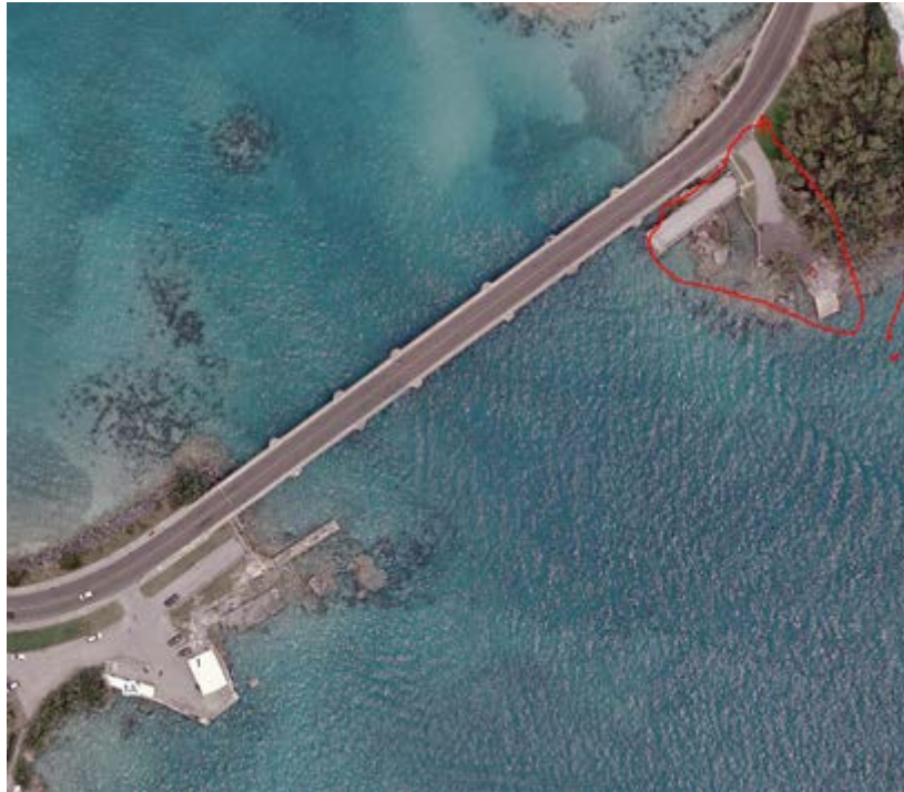
Figure 3. Laydown area available (WEDCo)
