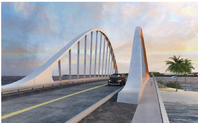
Figure 2. Steel tied arch for Longbird Bridge Replacement
