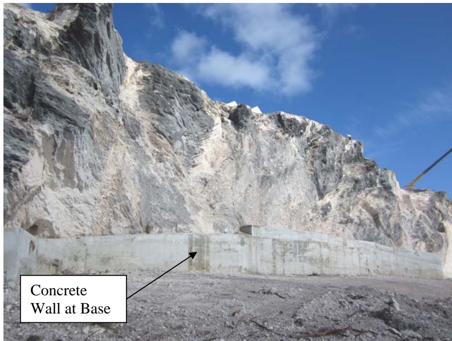
Photo 2: Central Part of Shore Cliff
